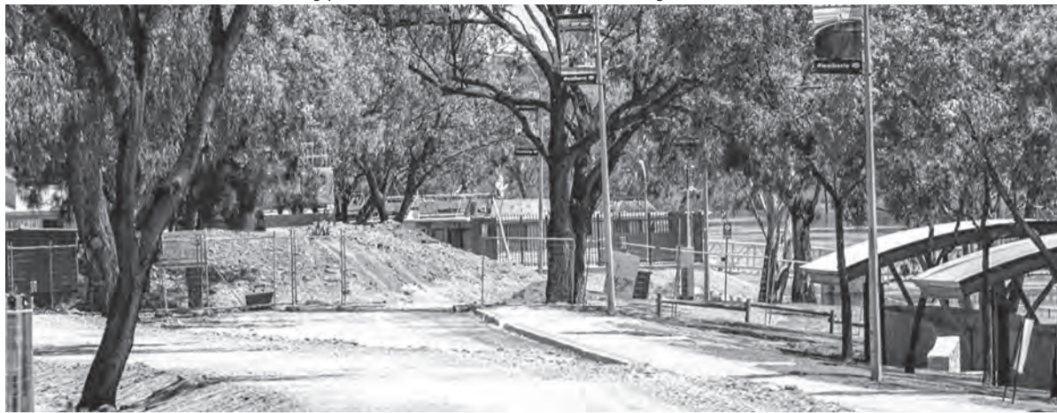
The levee bank that has been extended along the Waikerie riverfront is part of Loxton Waikerie council's defensive strategy against a flood scenario of 250GL a day. PHOTO: Paul McCormick
