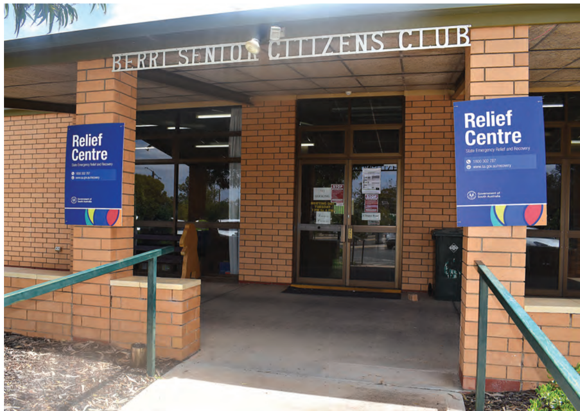
The first Emergency Relief Centre for the ongoing flood event opened at the Berri Senior Citizens Club building on Crawford Terrace yesterday. PHOTO: Alexandra Bull
