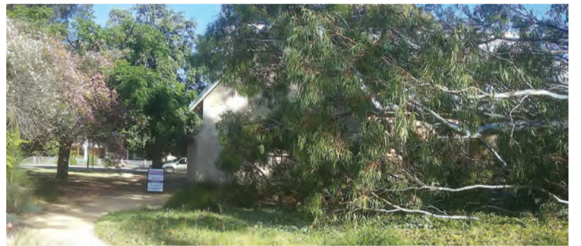
CLOSE CALL FOR CHURCH: The Renmark Anglican Church, on James Avenue, avoided potentially major damage after a gum tree fell due to flood waters last weekend. PHOTO: Ian Kent
