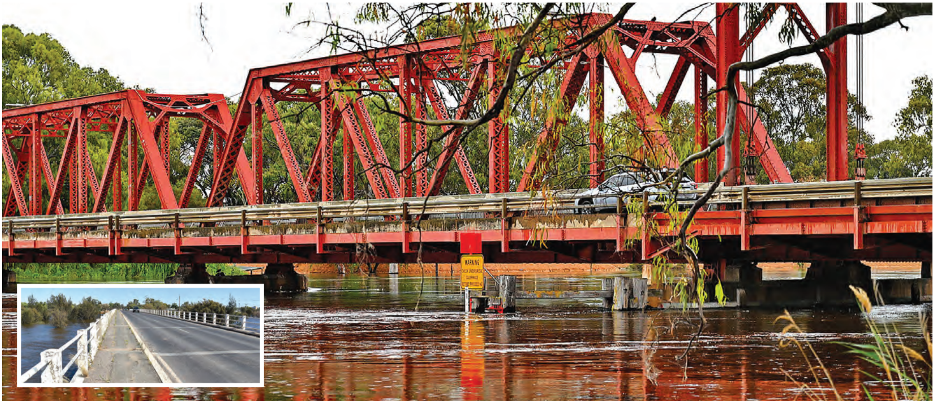
Exclusion zones have been introduced around Paringa Bridge and Ral Ral Bridge (inset) due to insufficient clearance. MAIN PHOTO: Grant Schwartzkopff
