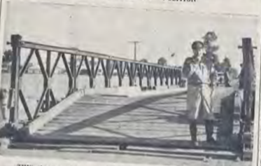
THIS shot was taken shortly after the Army had completed its rapid construction of the heavy bridge on Ball Hall Avenue, standing steady in the face of a great deal for the Renmark flood effect, Mr Frank Tisdale.
