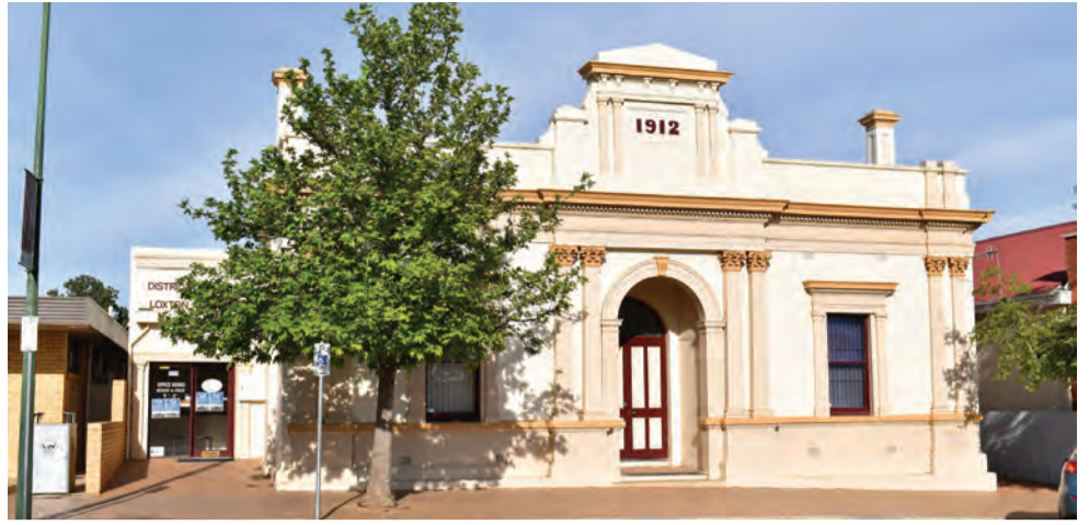
Proposed designs have been presented to Loxton Waikerie councillors for a new library, VIC and public amenities at the Loxton Institute building (pictured). PHOTO: Stephanie Thompson
